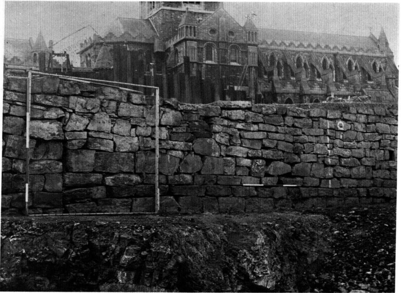
Fig 109 Wood Quay, Dublin: stone wall c 1100, with Christchurch Cathedral to north
